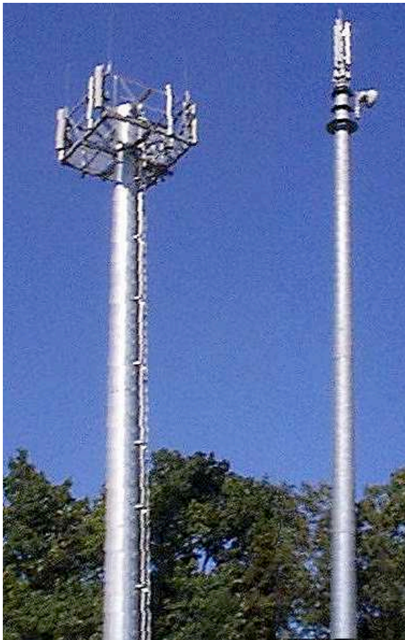
Figure 6: The difference in visual impact between base stations using space diversity (left) and polarization diversity (right)
