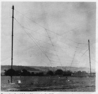
Even simple wideband log-periodic HF antennas are large and difficult to erect quickly in the field. The need for tall supporting masts is a major problem.
